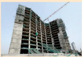
Tower Area view - 19th Floor slab casting work in progress
